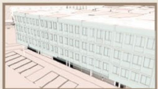
EGG-CRATE SHADING Vertical and horizontal shading elements as shophouses' facade suitable for Malaysia's hot climate
